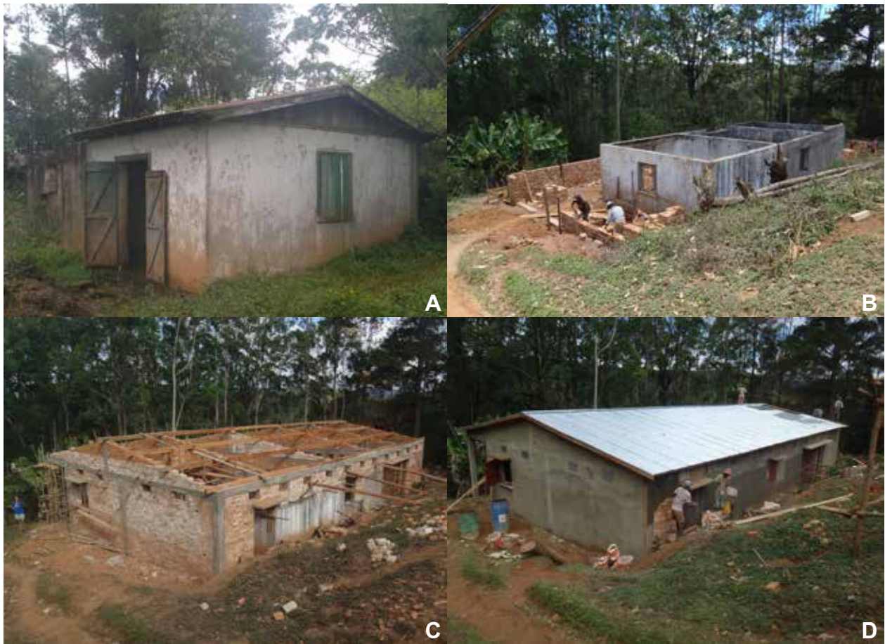
Figure 1. The facility was constructed between November 2010 and March 2011 from the foundations of an old abandoned forest station. A) Original abandoned building in January 2009. B) Facility construction November 2010. C) Facility construction December 2010. D) Facility construction January 2011.
